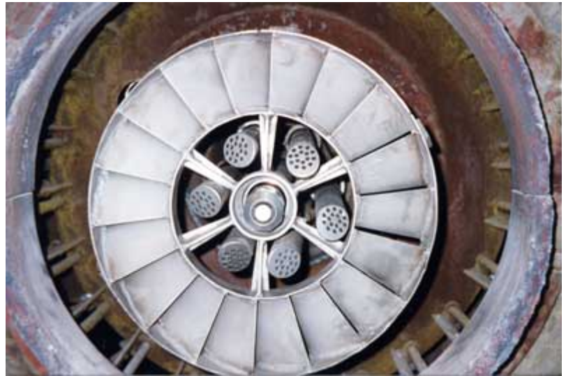
View of Burner Throat Showing COEN Flame Stabilizer, Gas Injectors and Oil Atomizer
