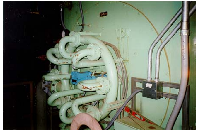
Fig. 1 Coen DAF-42 Low NOx Burner
